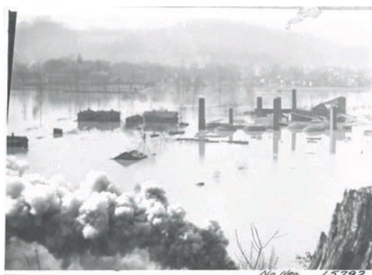
Figure 22 — Historical photograph of Cumberland River flood, 1939, Burnside, Kentucky (US Army Corps of Engineers)
