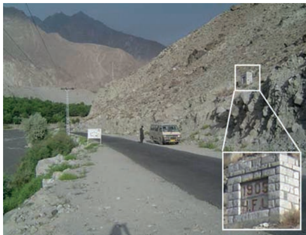
Figure 24 — High flood level of 1905 flash flood event in Khizer River, Gilgit-Balistan, Pakistan (Photo: Markus Zimmermann, August 2006)
